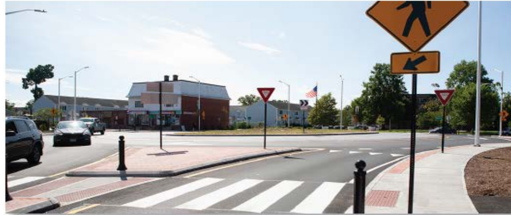
Six Corners Roundabout, Hancock Street/Walnut Street/Ashley Street/ Alden Street, Springfield
